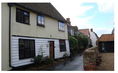
Figure 27 Vernacular materials including painted render, weatherboarding, clay tiles and pantiles and red brick boundary walls
