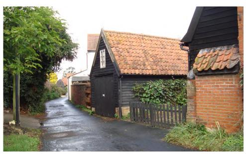
Figure 28 Timber weatherboarding and clay pantiles on outbuilding with picket fencing
